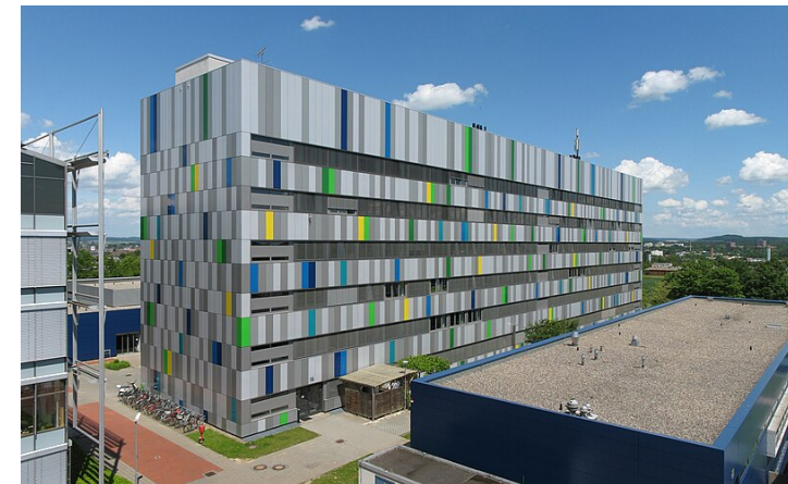
Physics Building, Photo: Klaus Foehl
