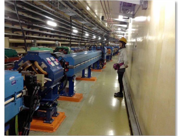
HER Warm Dipoles in Tunnel at KEK.
