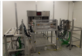
Pedestal comparison before and after HS Commissioning - Module W09_IB
