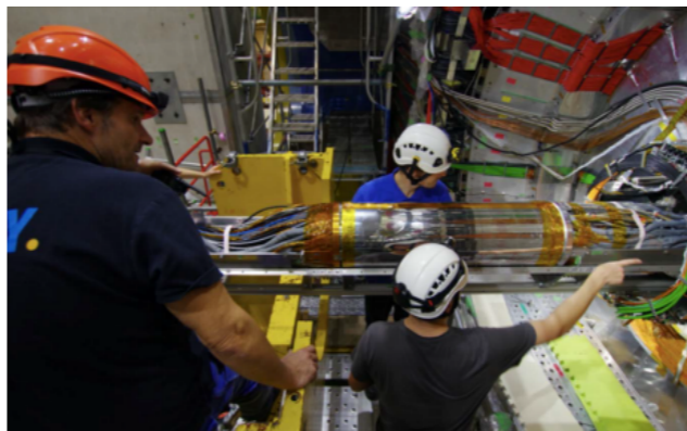
Installation of VXD
