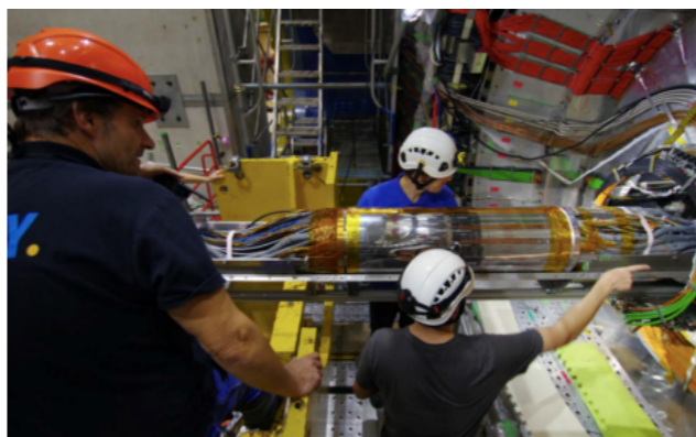
Installation of VXD
