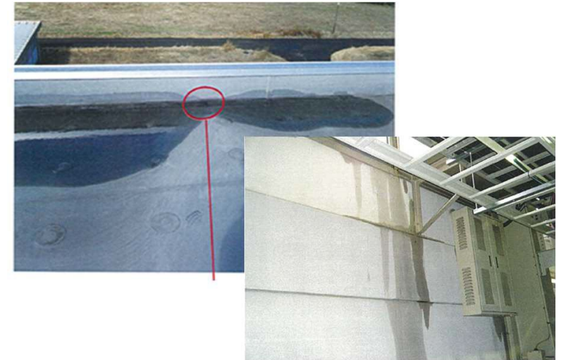
Leakage of roof of power supply buildings
