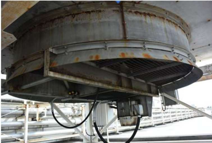
Erosion of Klystron cooling towers
