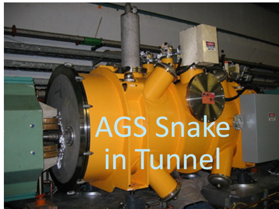
Figure 44: View of the BNL Manufactured Superconducting Snake Module Installed in the AGS Tunnel. The AGS Snake superconducting coil structure is housed in a standalone cryostat that is sandwiched in an otherwise normal conducting magnet accelerator lattice. This system uses local cryocooler based cooling along with a low heat leak support structure.
